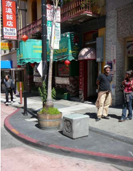
Bulbouts in Chinatown expand the pedestrian realm.
