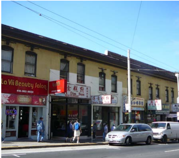
The existing building holds two beauty salons, a dim sum restaurant and noodle shop, a food distributor, and a real estate agent, among other uses, as well as over a dozen housing units upstairs.
